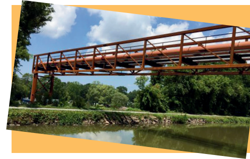
Sample Pipe Bridge over the Canal
